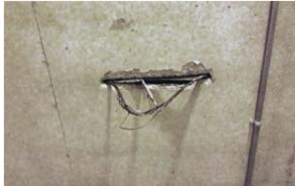
Figure 4-1: Eruption of PT Tendons caused by Corrosion Failure (Vector Corrosion Technologies, 2019)
