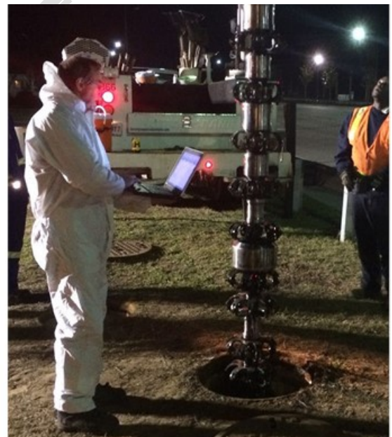
Figure 5 Image showing SeeSnake being lowered into the pipe through a manhole
