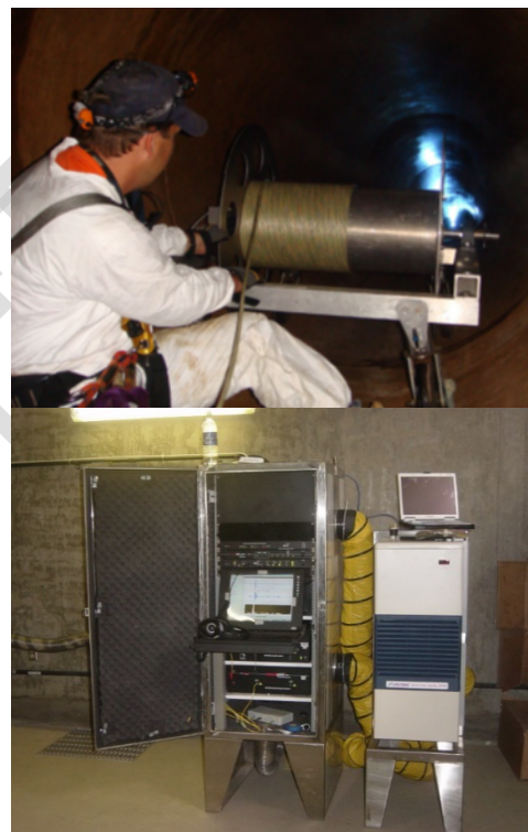
Figure 1. Installation of a fiberoptic system inside a pipe (top); Data acquisition system (bottom)
