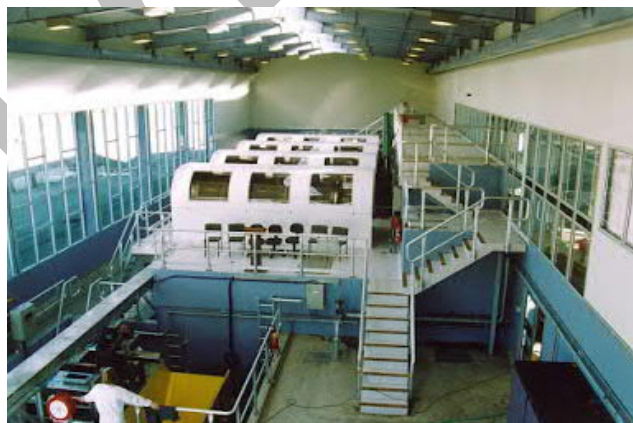
Photo 1 Napier Wastewater Treatment Plant Milliscreen
