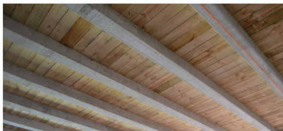
Exposed Stalhton Rib & Infill
